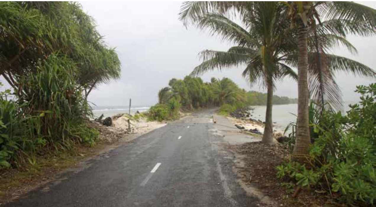
Most narrow path of Funafuti main atoll of Tuvalu.
