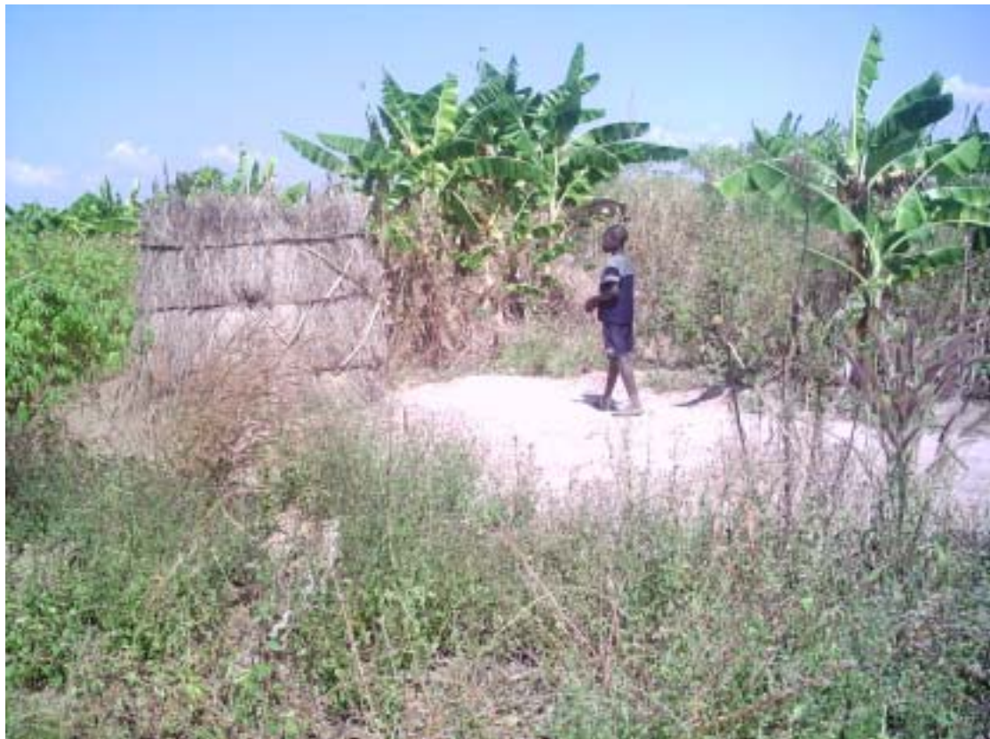
Family Pit Latrine, Cazombo, 2004
